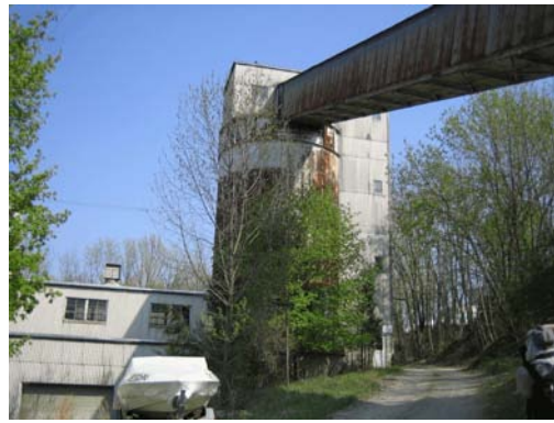
upper mine with conveyor belt
